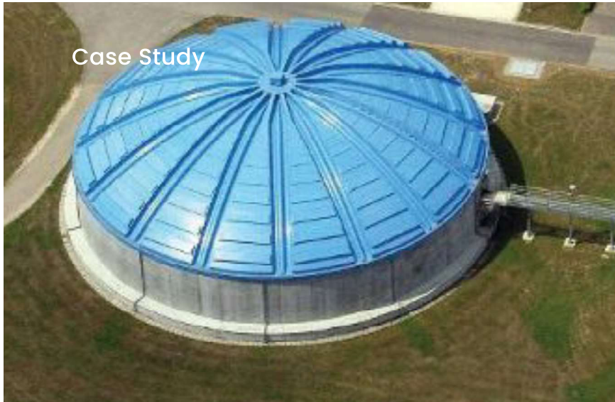
A fiberglass-reinforced plastic dome covering system spanning 120 feet.
