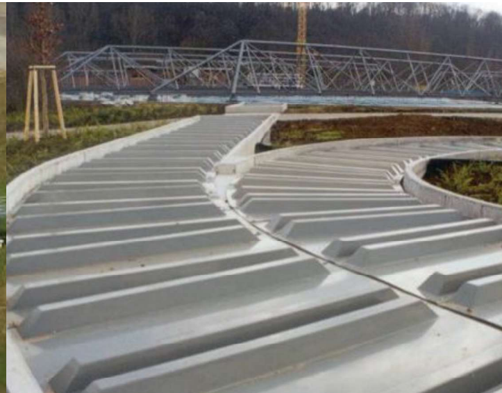
A single-shell covering with profiled elements.
